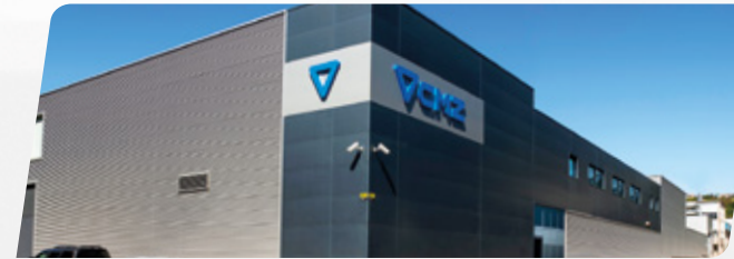
CNC lathes Assembly plant 5,500 m2 | Zaldibar – Spain
