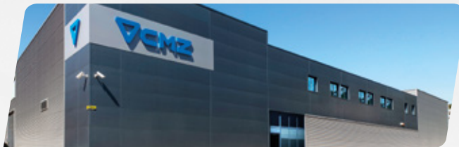
CENTRAL SERVICES | TECHNICAL ASSISTANCE SERVICE Zaldibar – Spain
