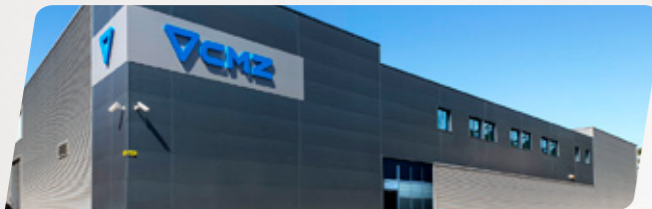
CENTRAL SERVICES | TECHNICAL ASSISTANCE SERVICE Zaldibar – Spain
