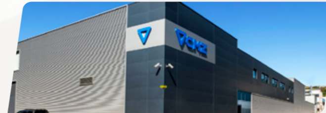
CNC lathes Assembly plant 5,500 m2 | Zaldibar – Spain
