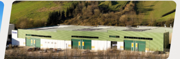
CNC lathes Assembly plant 10,000 m2 | Mallabia – Spain
