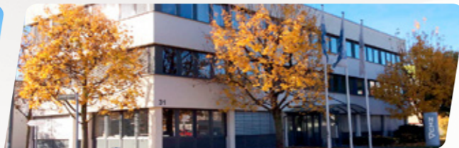
COMMERCIAL OFFICE | TECHNICAL ASSISTANCE SERVICE Stuttgart – Germany
