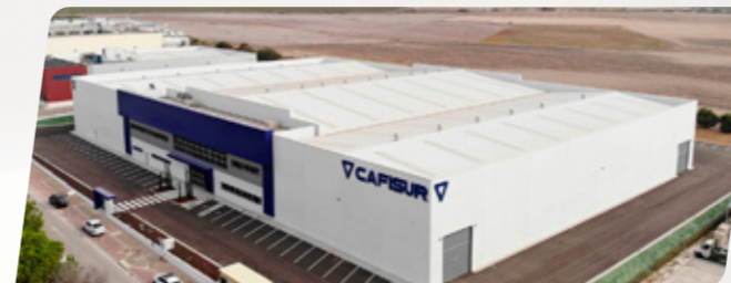
Sheet metal plant 15,000 m2 | Cádiz – Spain
