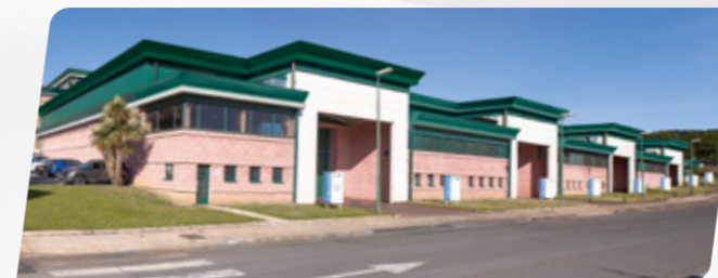
Machining plant 4,900 m 2 | Elorrio - Spain
