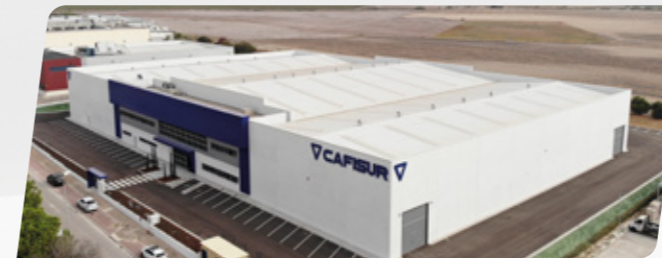
Sheet metal plant 15,000 m 2 | Cádiz - Spain
