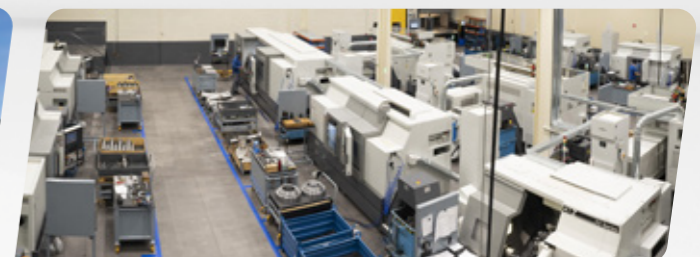
Machining plant 2,000 m 2 | Elorrio - Spain
